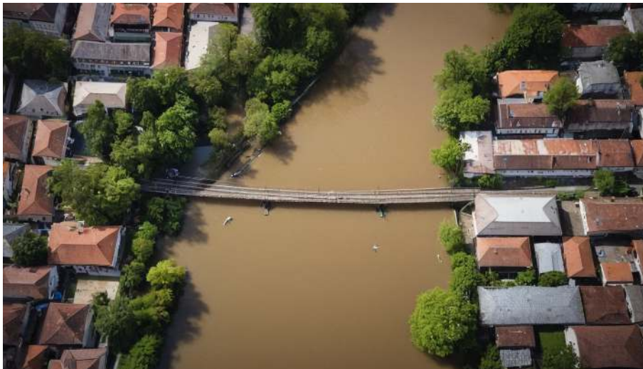
Figure 82. "prompt": "<|system|> You are a Stable Diffusion prompt generator.<|user|> Come up with a description of a flooded river at night on a Austrian town, trapped cards, damaged bridge. <|assistant|>" [image generated by ATOS]
